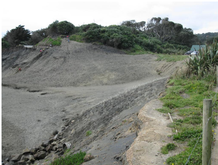
Newly excavated and reshaped area 2009
